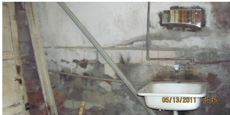
Monitoring undertaken in May 2011
