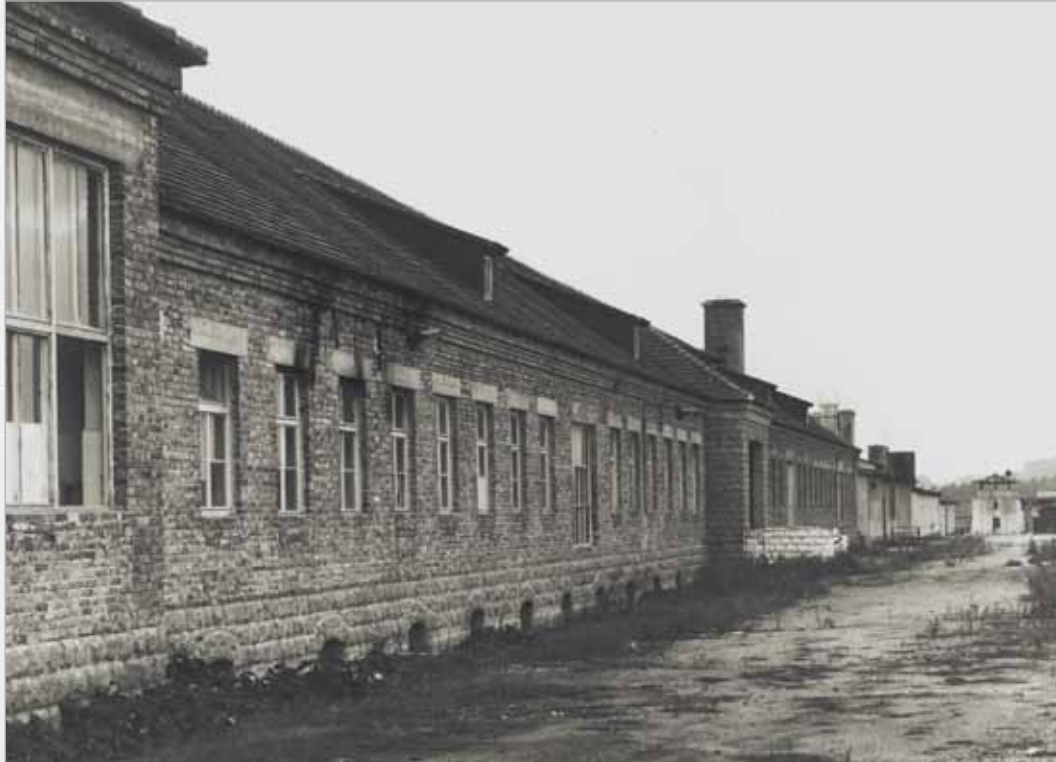
This photograph taken in 1946 shows the historical condition of the building without plastering (© Photograph Archive of the Mauthausen Memorial, BHÖ Collection).
